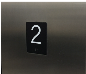
Elevator Door Jamb: Example of Tactile / braille floor designation signage.
