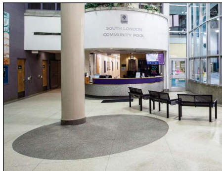
Where a structural column / support may be within an accessible route, a colour contrasted floor surface at the base helps identify its location to prevent a potential bumping hazard.
