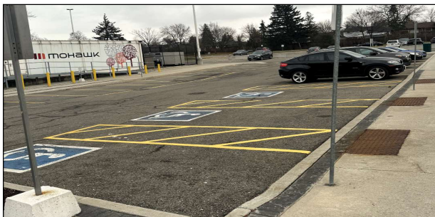
Accessible parking spaces with access aisle and curb ramp.
