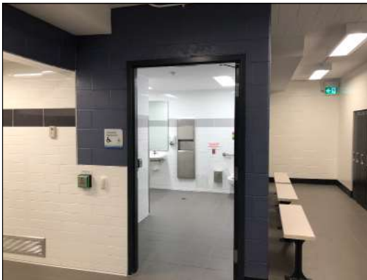
Example of a universal washroom integrated as part of an accessible change room.
