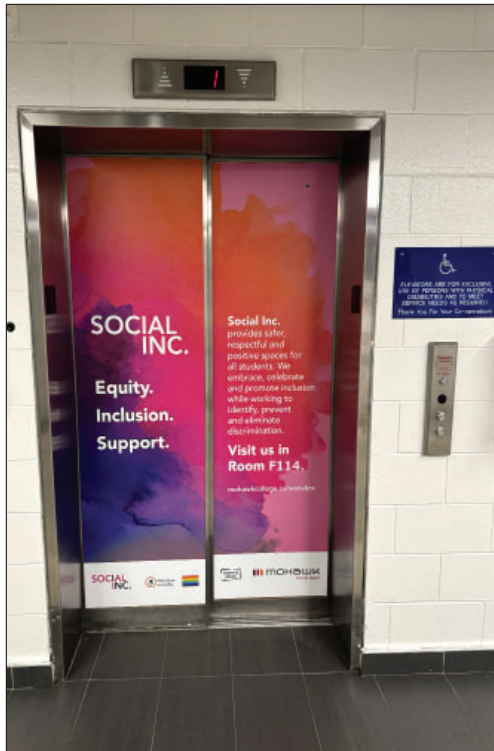
View of an accessible elevator and typical features in lobby.
