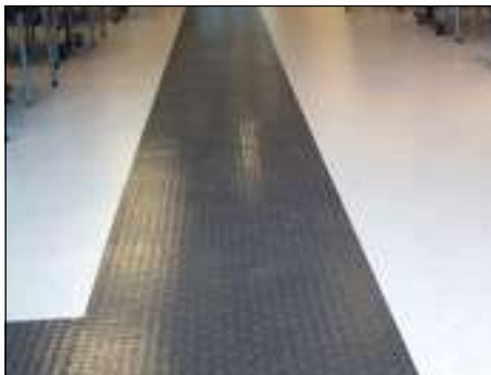
Example of tactile floor surface to guide users with vision loss (Best Practice).
